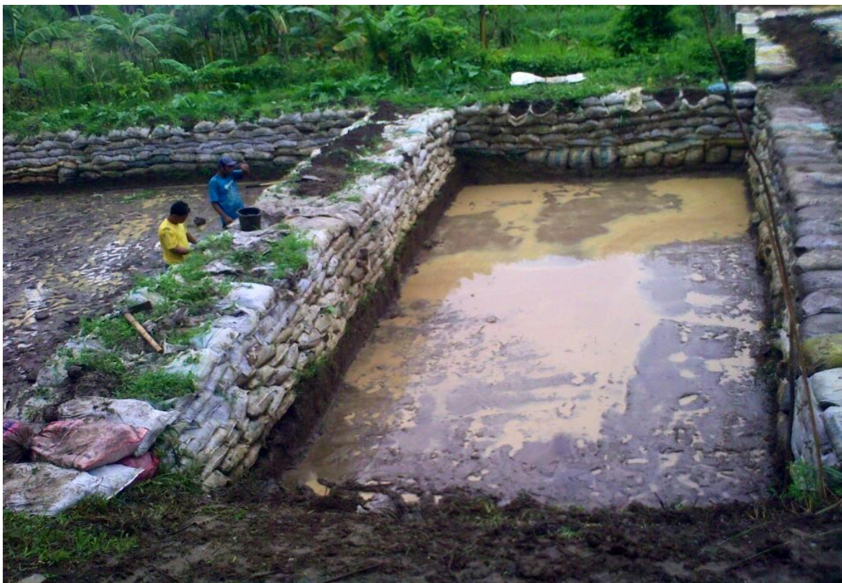
Fig. 4. In wetland-based aquaculture systems, fish ponds can be created by constructing 90-degree embankments using sandbags for structural support and water retention.
