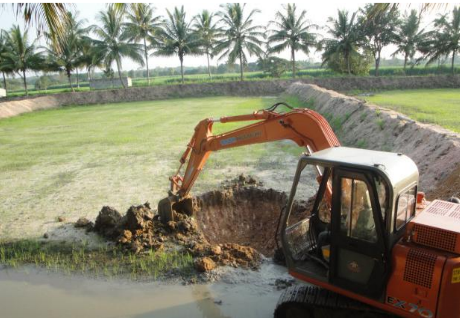
Fig 6. In waterlogged areas, constructing a step-up pond by excavating soil only along the periphery by making a trench and subsequently leveling it upon completion can reduce construction costs by up to 60%.
